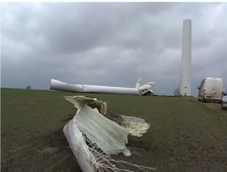
Figure 4: collapse of a windmill February 2007
