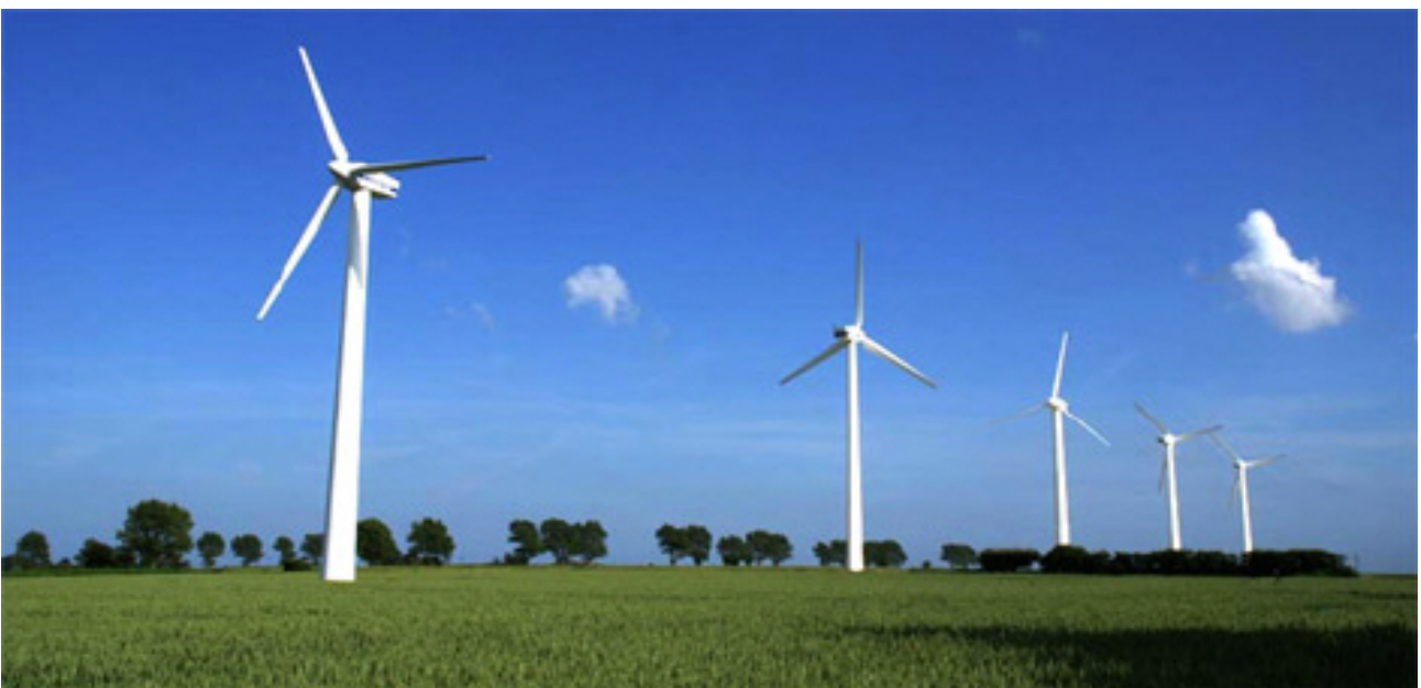
Figure 6: impact of megaturbines on the landscape
